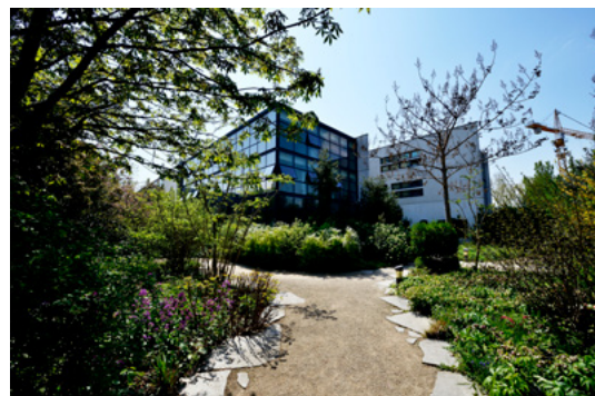
The Buisson building
