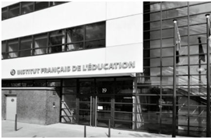
FERDINAND BUISSON BUILDING
